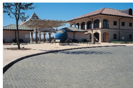
The LEED system gives credits to the runoff and pollution reduction characteristics of permeable interlocking concrete pavers.
